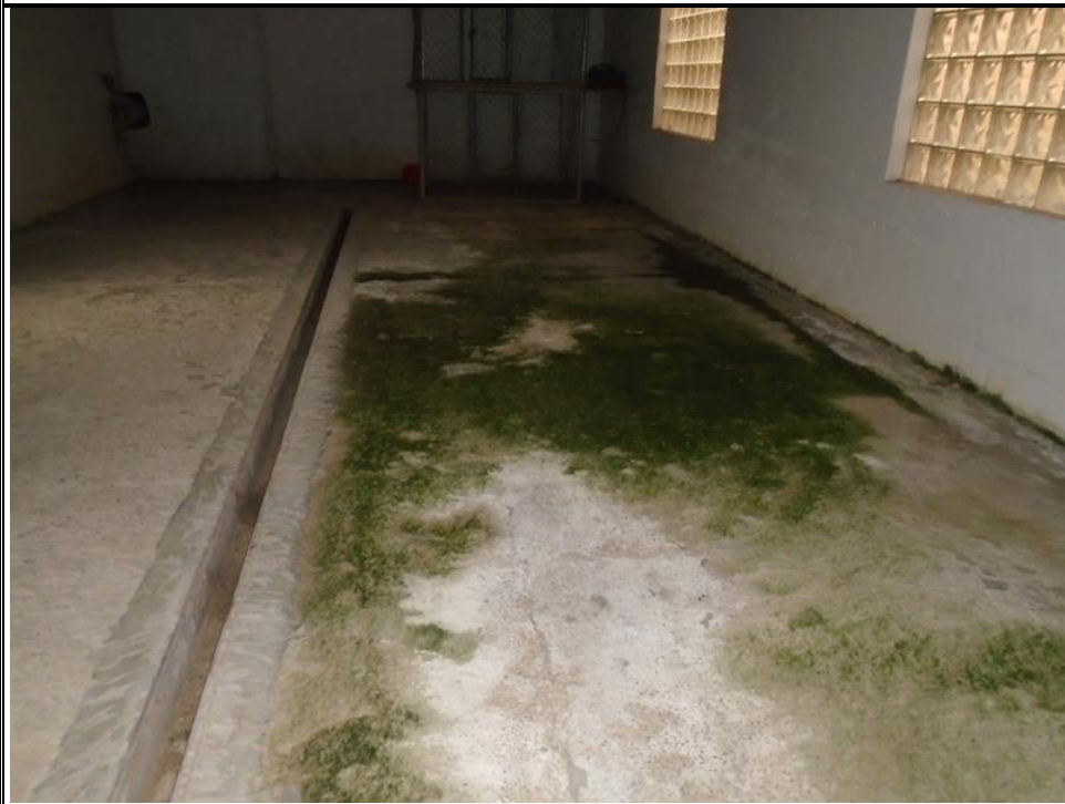
REAR ROOM – TRENCH DRAINING AND MOLD
