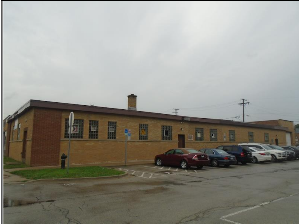
EAST ELEVATION – 9150 W. GRAND AVENUE AND MUNICIPAL PARKING LOT
