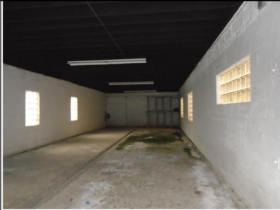
REAR ROOM AT NORTHWEST ELEVATION
