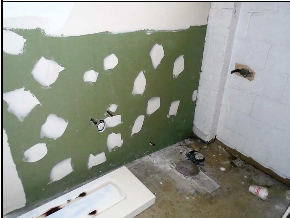
WASHROOM WITHOUT PLUMBING FIXTURES
