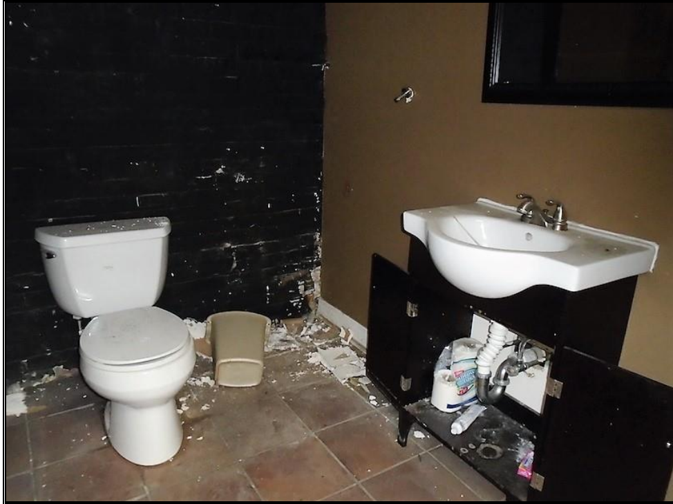
WASHROOM WITH PLUMBING FIXTURES
