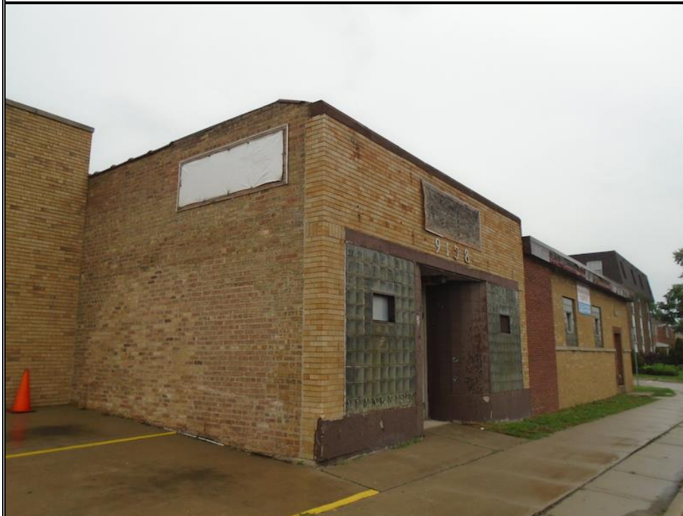
SOUTHWEST ELEVATION – 9158 GRAND AVENUE
