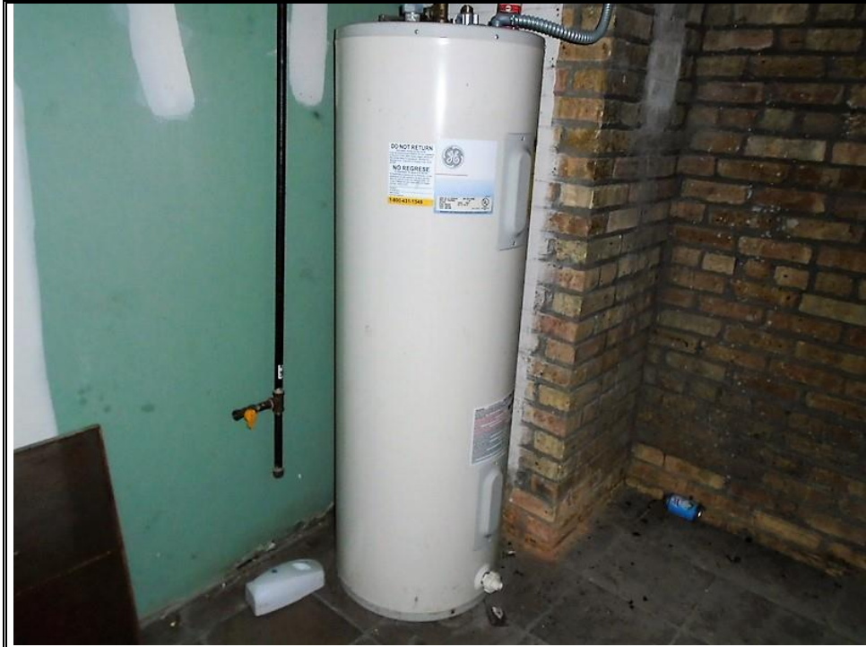
WATER HEATER ROOM
