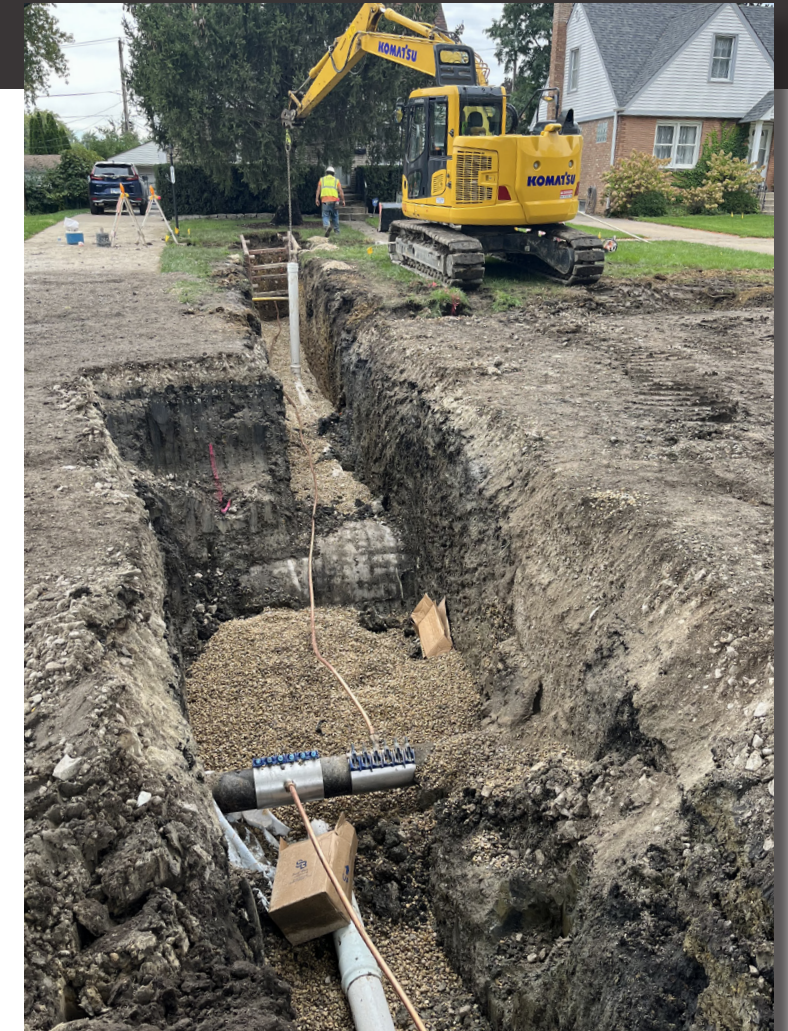
Along with the installation of new water mains, lead service lines were replaced to ensure that properties had safe access to clean water.
