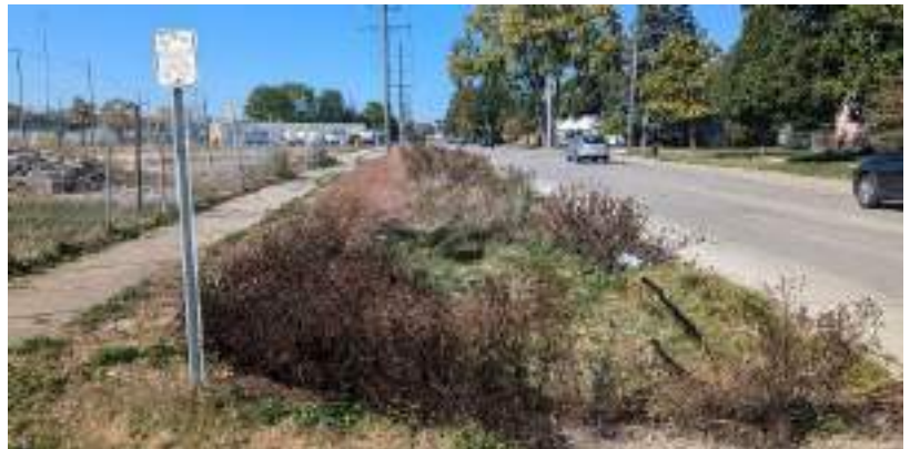
Figure 20: Rain Garden Implemented through MWRD Program
