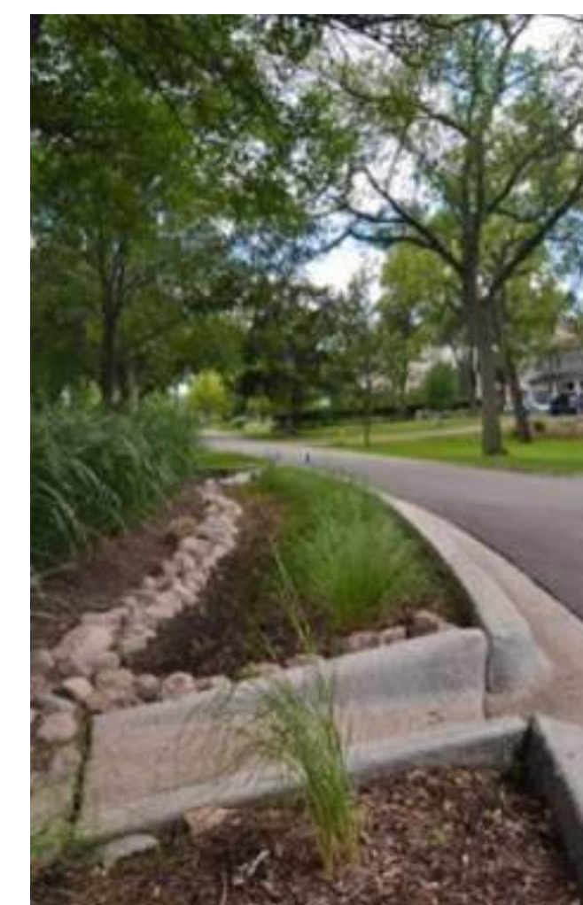
Bioswale planting strips along Scott St and Fullerton Ave
