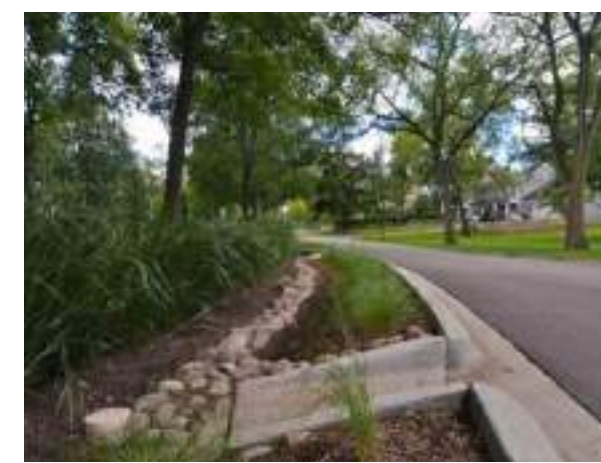
Bioswale planting strips, Houston St looking North
