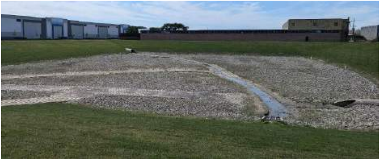
Figure 3: Stormwater Detention Pond at Addison Avenue and Wolf Road
